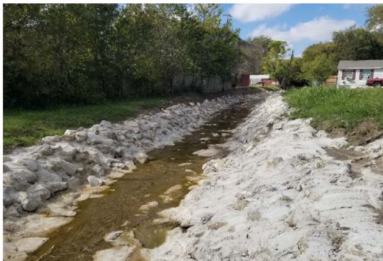
Picture of the concrete rock rip-rap placement
