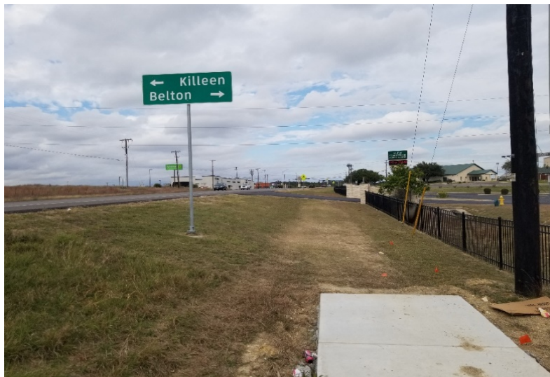
Area of construction for the sidewalk.
