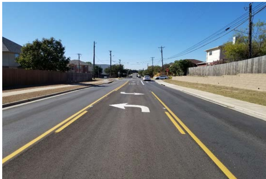
One of the completed streets in the FY 2019 Miscellaneous Street Projects.
