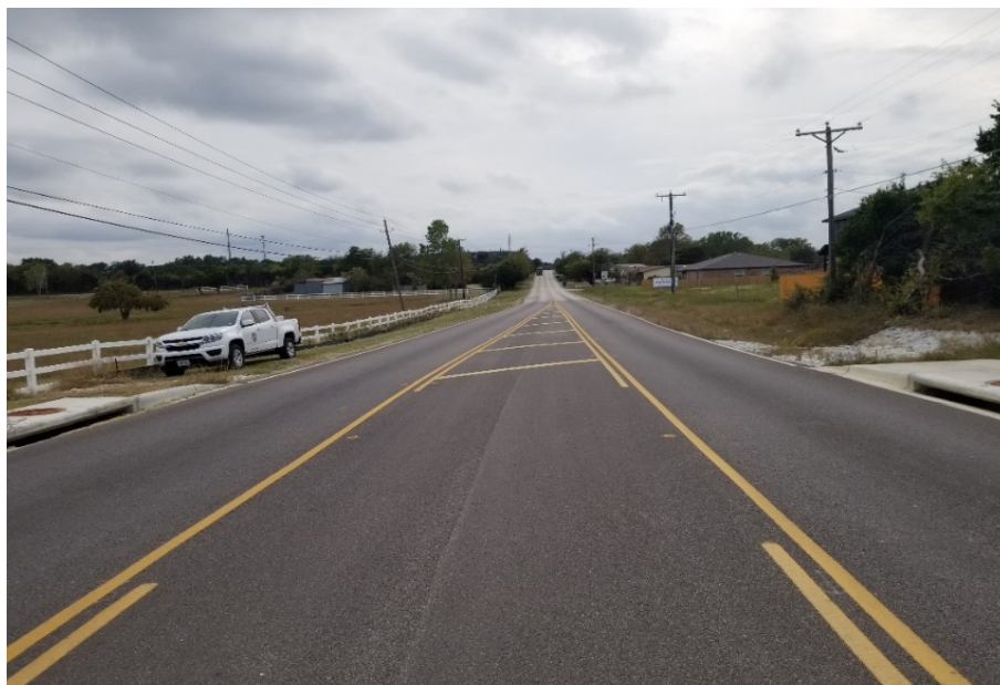
A completed Warrior's Path Phase 1 with what will be Warrior's Path Phase 2 in the horizon.
