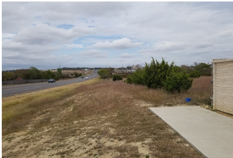
Area of construction for the sidewalk.
