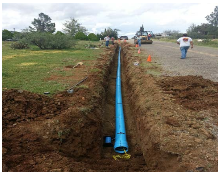
Example of the installation of a waterline.
