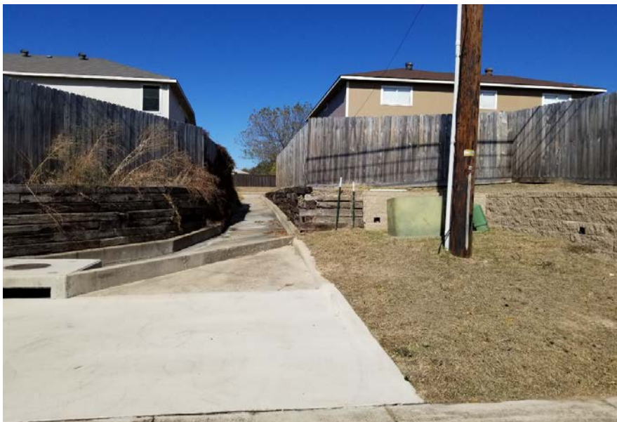
Site of the Drainage Flume Reconstruction Project.
